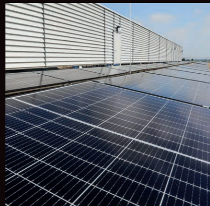
Rooftop solar PV project coming soon
