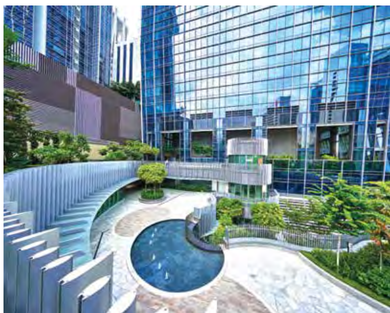
▲ Frasers Tower • Singapore
